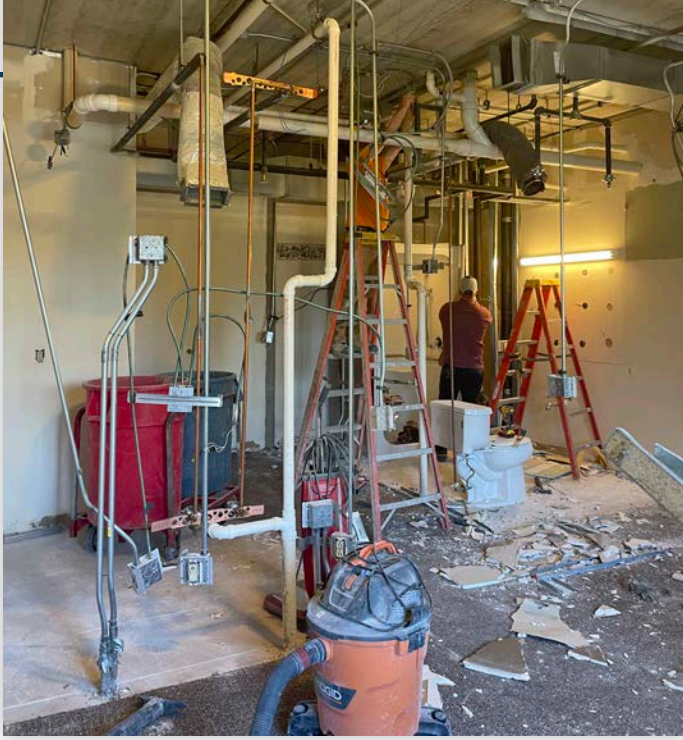
The first phase of renovation to the existing units involved demolition of interior walls to expand the footprint of the floor plan.
