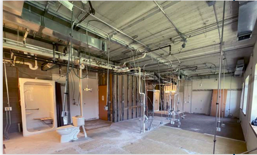
The first phase of renovation to the existing units involved demolition of interior walls to expand the footprint of the floor plan.
